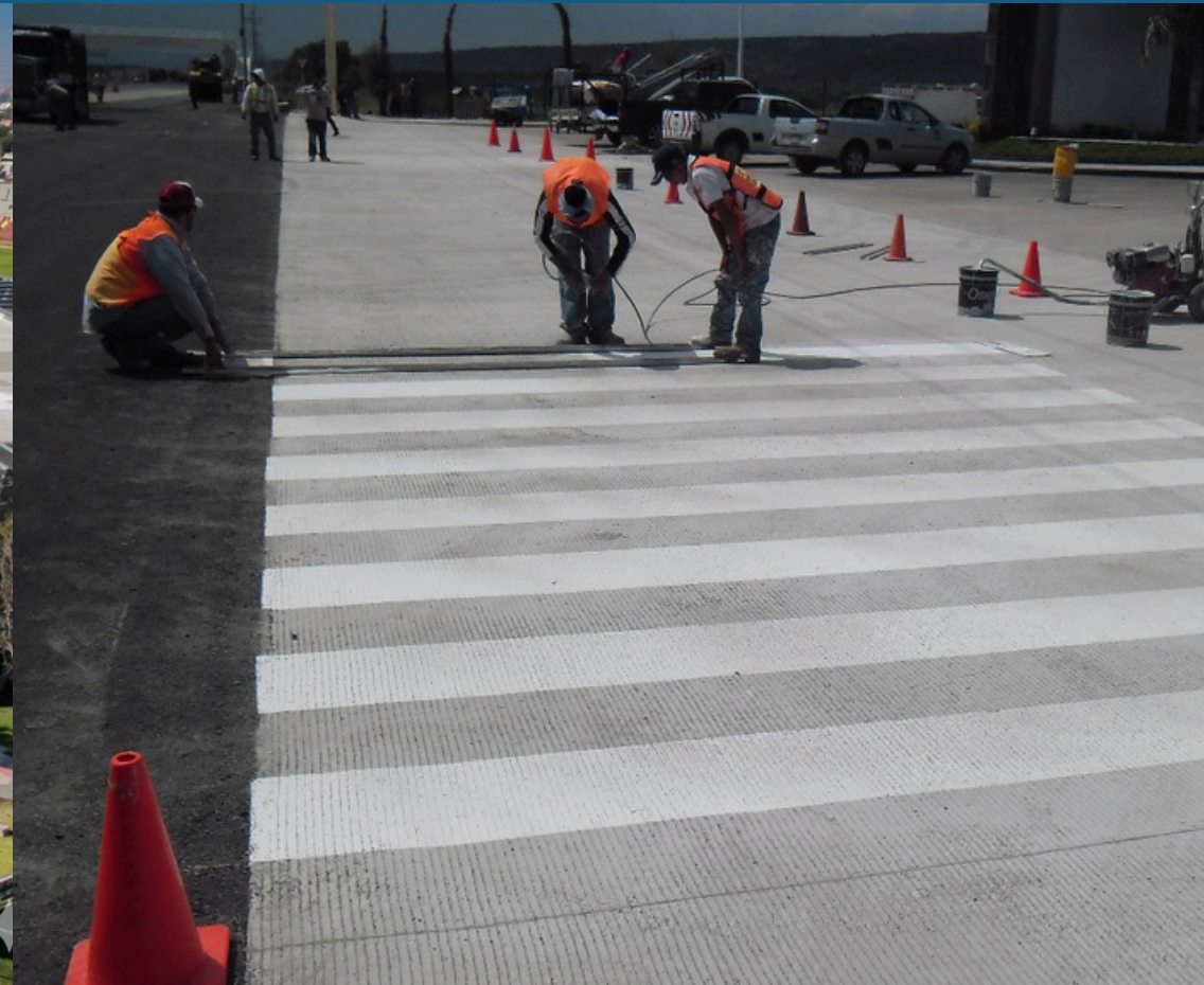
ROADWORKS: Deceleration Lane for Access to AeroTech Industrial Park, State Highway No. 200, Municipality of Colón, Querétaro.
