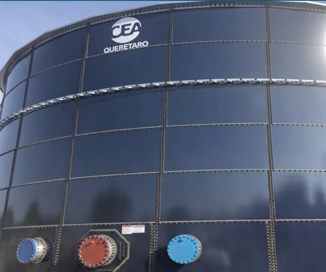
HYDRAULIC: Drinking Water Storage Tank, San Francisco - Arroyo Hondo Community, Municipality of Corregidora, Querétaro.
