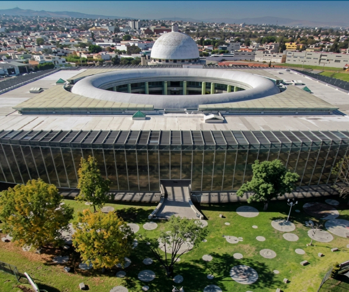
BUILDING: "Manuel Gómez Morín" Educational and Cultural Center of the State of Querétaro, Municipality of Querétaro, Querétaro.
